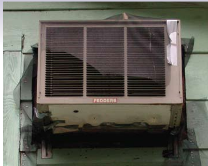
An inexpensive "one-way-door" made of screen often prevents bats from re-entering the house.
