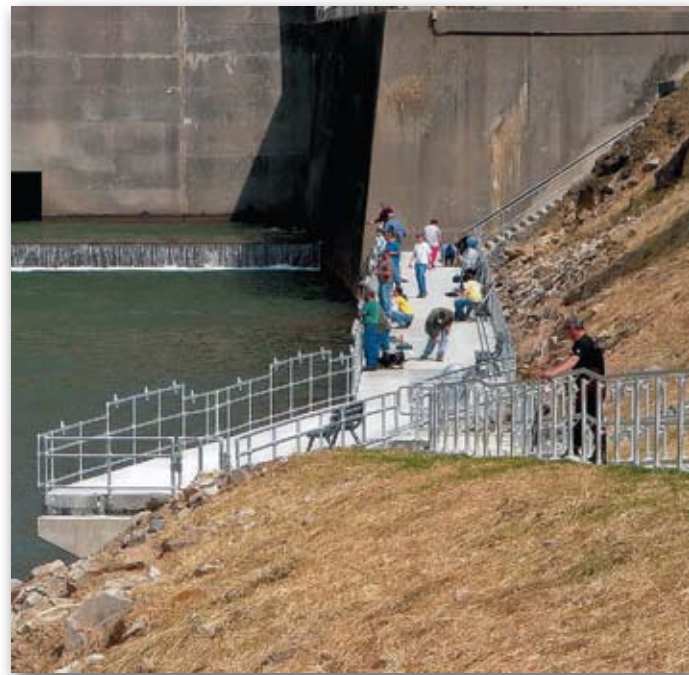
A new handicapped accessible pier provides access to the Sutton Dam tailwater.
