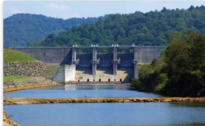
Burnsville tailwater is accessible by concrete anglers' path. (left side of photo)
