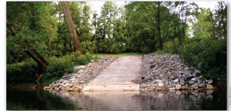
New boat ramp 3 miles north of Buckhannon built with pervious concrete to reduce water pollution.
