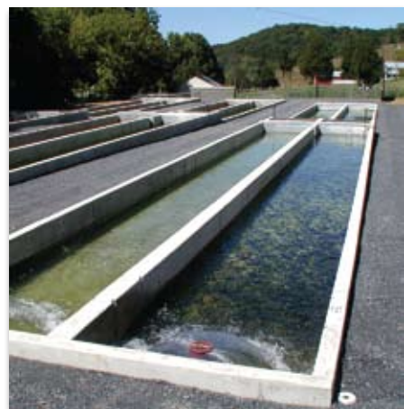
New raceways at Spring Run Hatchery.
